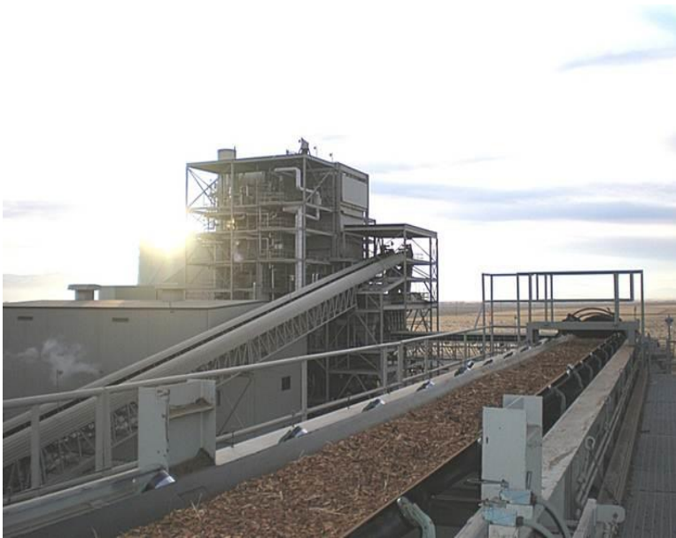
Honey Lake Power Plant in California
